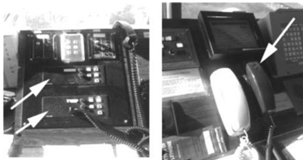
Fig. 2. Telephone handsets in the tower
